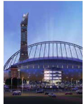
QATAR OLYMPIC & SPORTS MUSEUM QATAR
